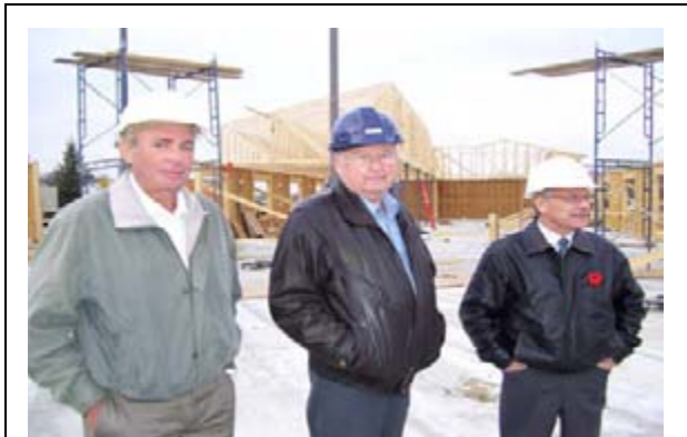
SHR Allan Daelick-VP of Operations Support, Grant See -Board member and Joe Kirwan-CEO make a visit to the construction site.
